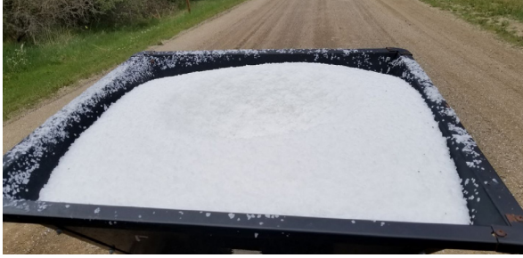
MAGNESIUM CHLORIDE APPLICATION ON RAILWAY AVE.
