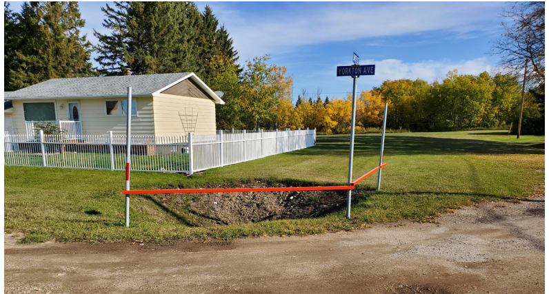
Barrier constructed Late Sept.
